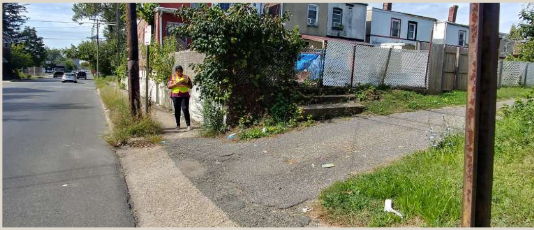
Figure 28. Poor sidewalk conditions north of Blane Alley.
