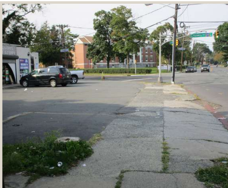
Figure 139. Continuous driveway access across sidewalk.
