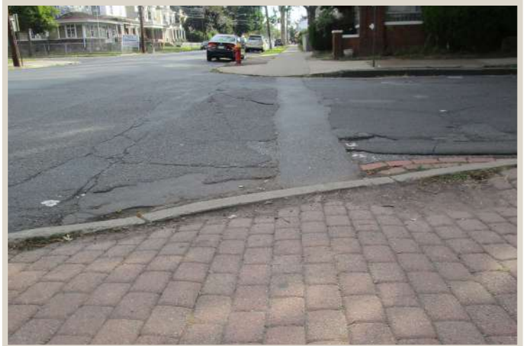
Figure 98. Missing crosswalk and non-compliant curb ramps.
