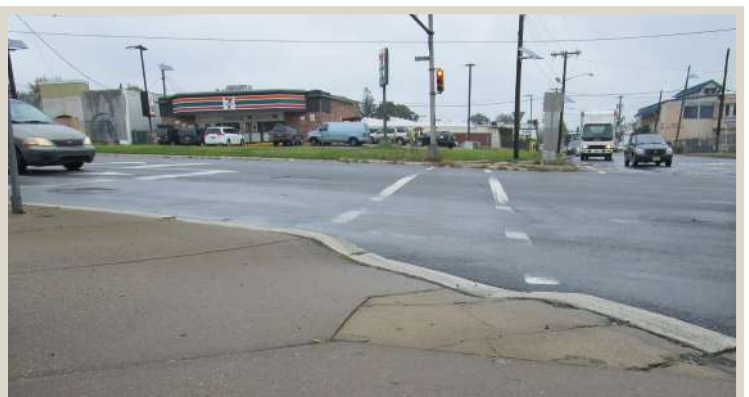
Figure 123. Non-compliant ramps and a turning radius that encourages high speed turns.
