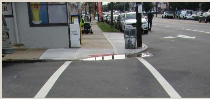
Figure 171. Water pooling at bottom of ramp.
