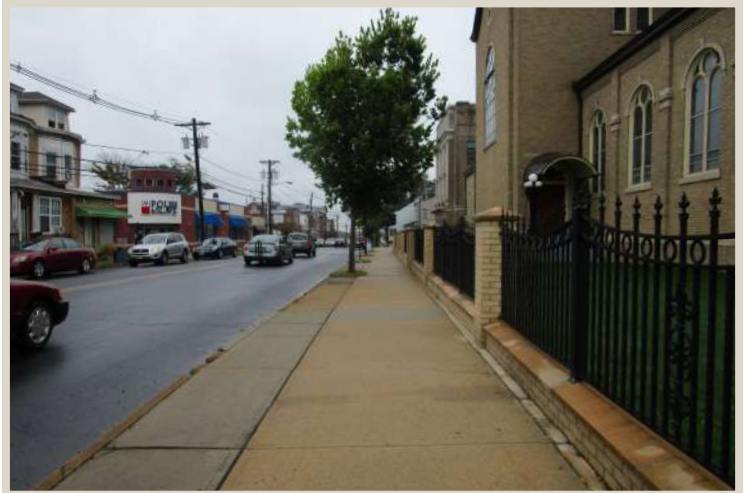
Figure 119. Sidewalk in good condition in front of St. Hedwig's Church.
