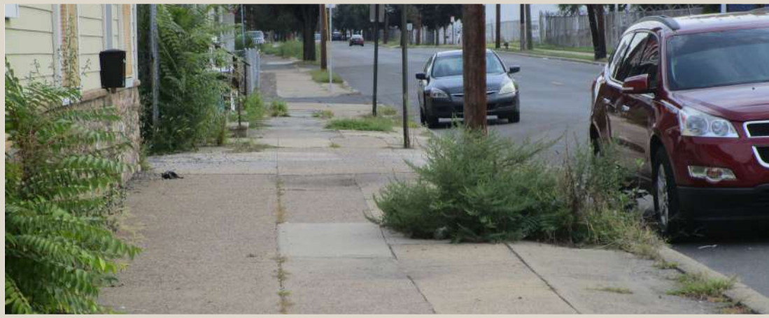
Figure 59. Cracked sidewalks and overgrown weeds.
