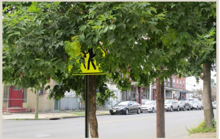
Figure 67. Mid-block crosswalk sign covered by overgrown tree.
