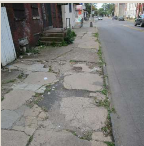
Figure 47. Significantly deteriorated sidewalk conditions.
