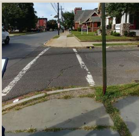
Figure 99. Missing curb ramps.
