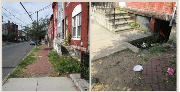
Figure 75. Gaps between varying sidewalk materials.
