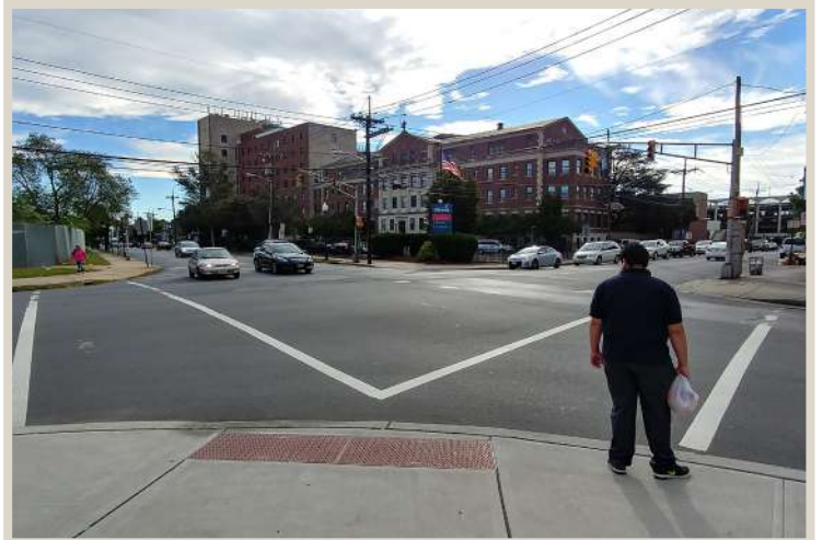
Figure 94. Only one ramp at intersection meets ADA standards.
