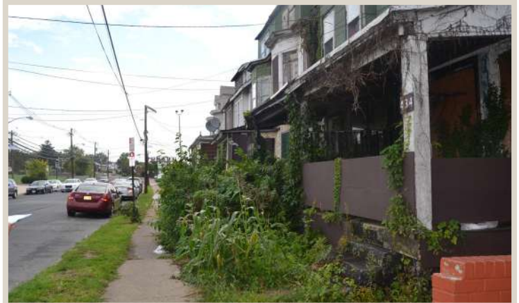
Figure 19. Overgrown vegetation on sidewalk.
