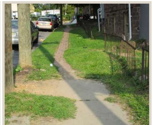
Figure 156. Sidewalk in poor condition.
