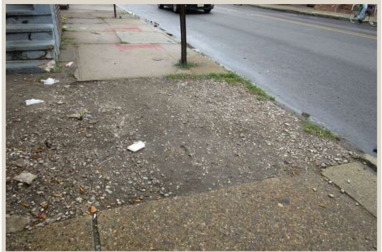
Figure 125. Sidewalk reduced to dirt and gravel.
