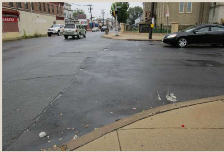
Figure 118. Severely faded crosswalk and stop lines.
