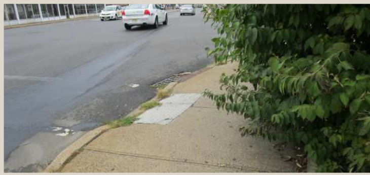
Figure 115. Non-compliant ramp with a bush blocking visibility.
