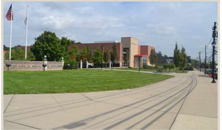
Figure 180. Wide sidewalks in excellent condition in front of the Martin Luther King Jr. School on Brunswick Avenue.
