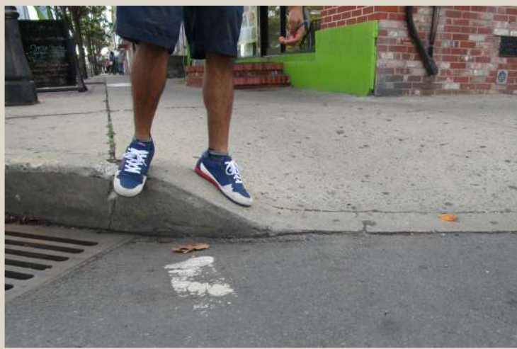
Figure 97. Curb ramp with a steep slope and missing truncated domes.
