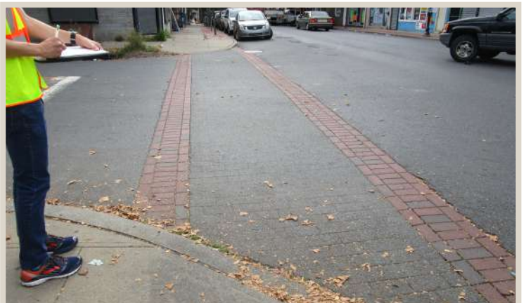
Figure 168. Crosswalk outlined in brick.
