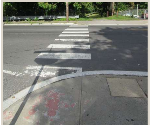
Figure 42. Continental crosswalk with faded ramps.
