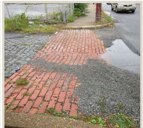
Figure 127. Missing curb ramps.
