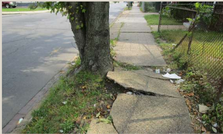
Figure 179. Dangerously uneven sidewalks along Pennington Avenue.
