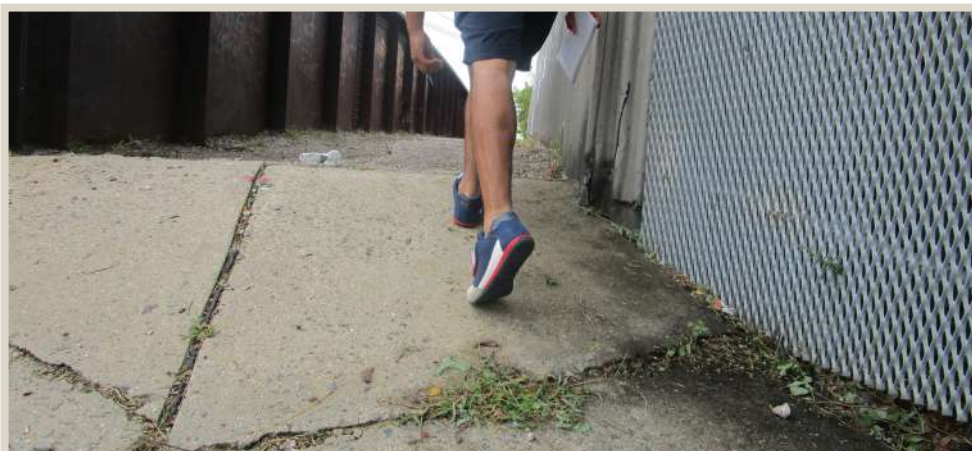
Figure 135. Steep incline along cracked sidewalks.
