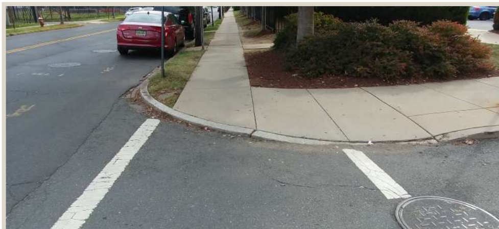
Figure 91. Non-compliant ADA ramps.
