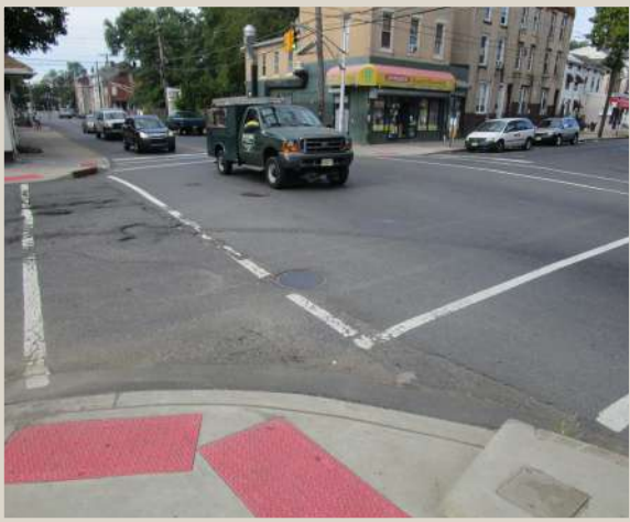
Figure 44. Updated ADA curb ramps, but missing pedestrian signals at Spring Street.
