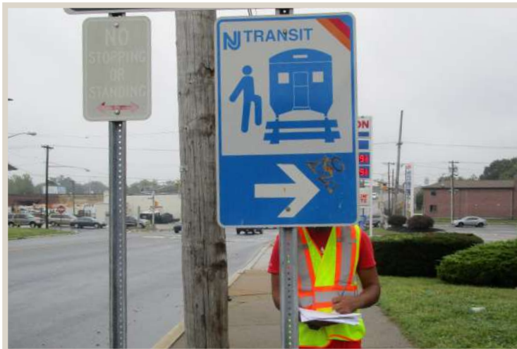
Figure 121. Faded and low-set signage.
