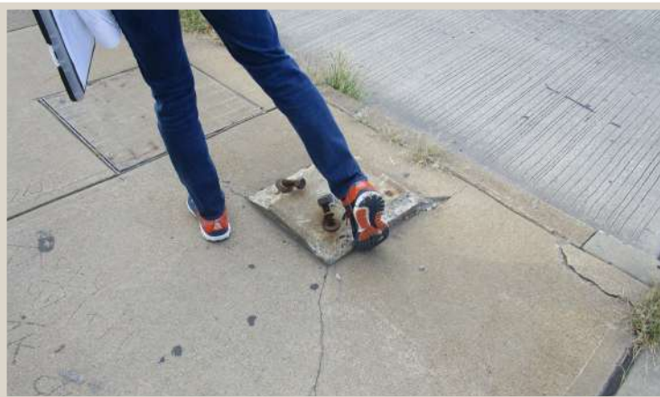
Figure 161. Tripping hazard along the sidewalk.
