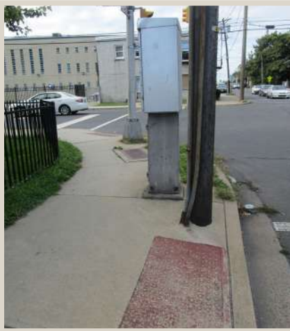
Figure 40. Electronic cabinet blocking pedestrians from drivers' sight.
