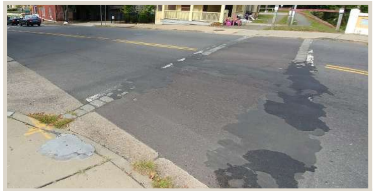
Figure 51. Asphalt-covered pavers along crosswalk.
