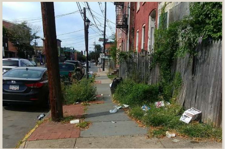
Figure 107. Sidewalk cluttered with litter and overgrown shrubbery.
