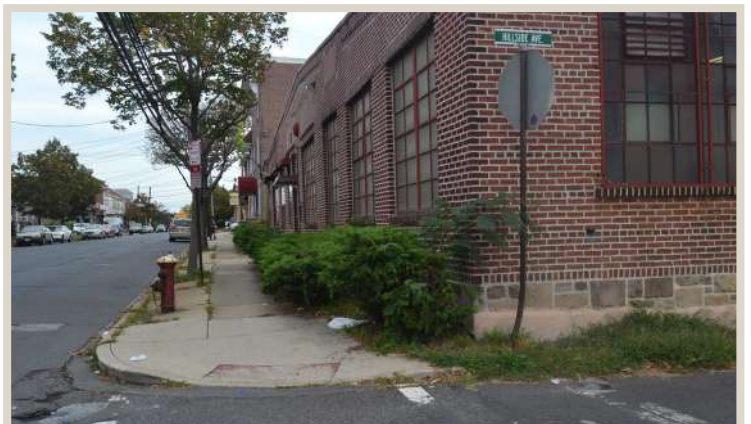
Figure 15. Building at corner of Brunswick and Hillside blocks sight lines for vehicles arriving at the stop sign.
