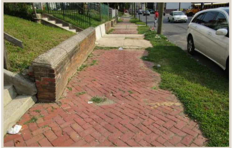
Figure 154. Sidewalk in poor condition.
