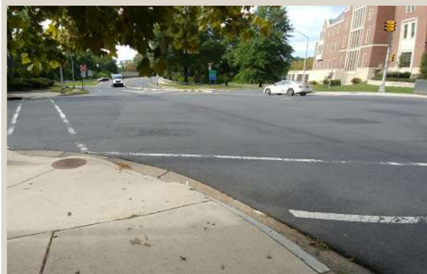
Figure 52. Large intersection at West State Street.
