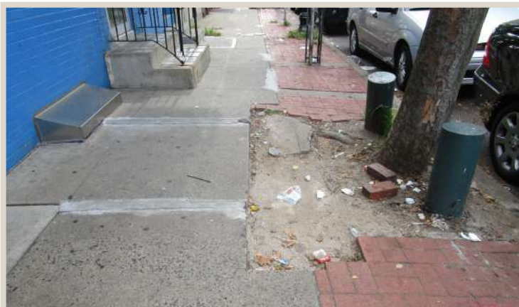
Figure 167. Sidewalk narrows due to unmaintained tree well and stairs.
