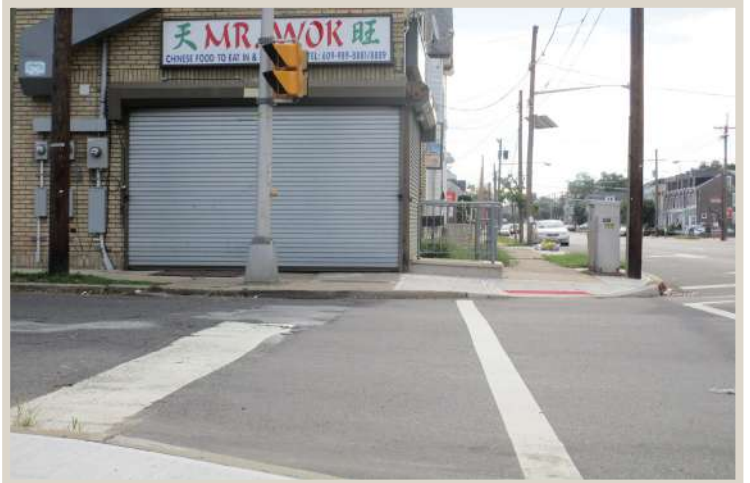
Figure 170. Misaligned pedestrian signal.
