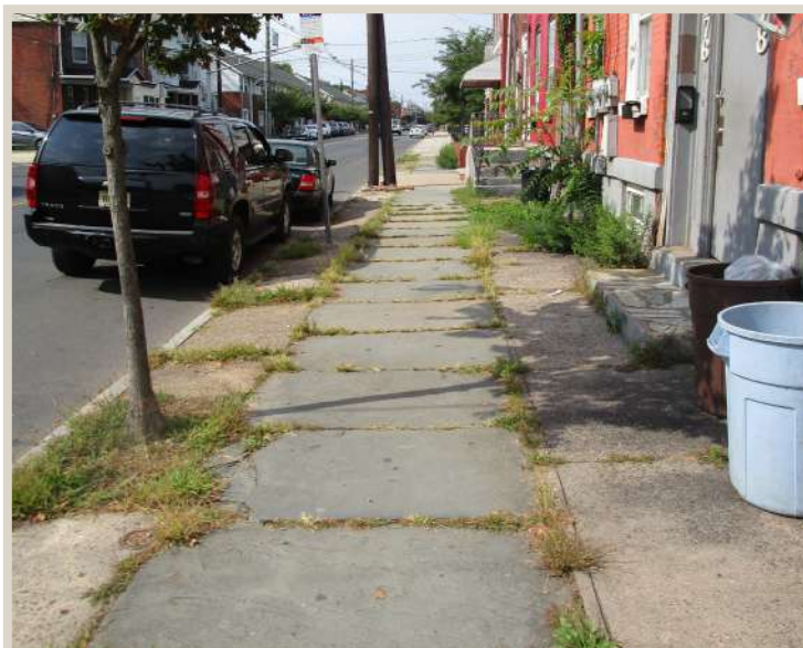
Figure 73. Vegetation growing between sidewalk panels.
