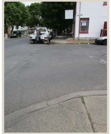
Figure 60. Missing curb ramps.
