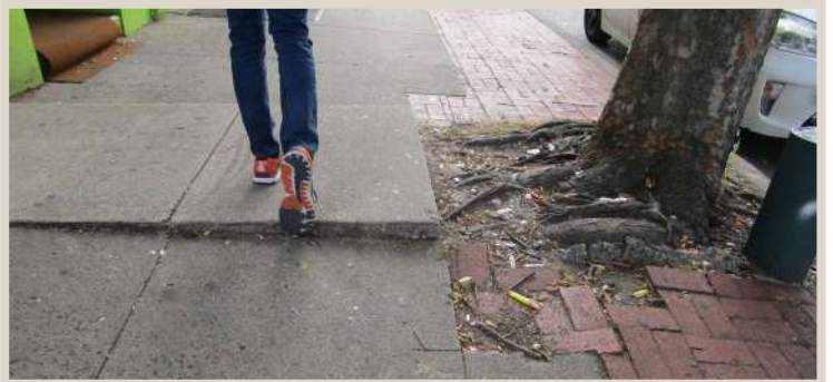
Figure 166. Raised sidewalk causes a tripping hazard.
