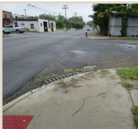
Figure 130. Missing curb ramps.
