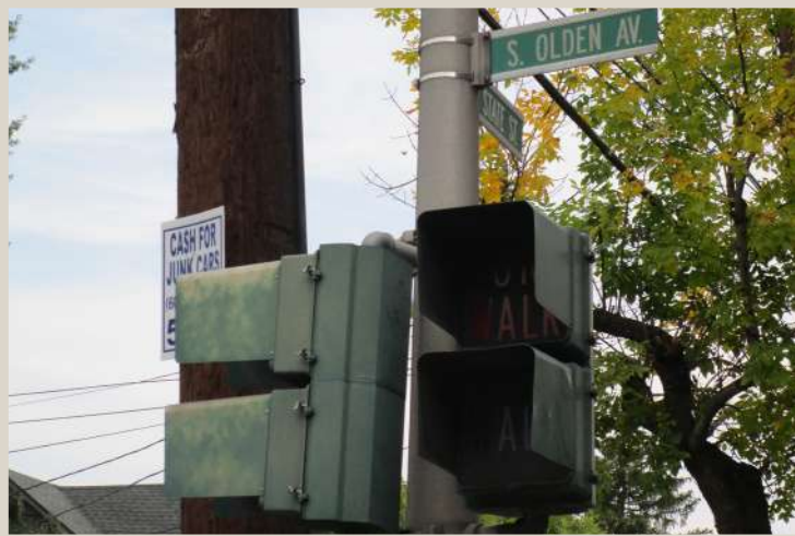
Figure 62. Dim and outdated pedestrian crossing signals.
