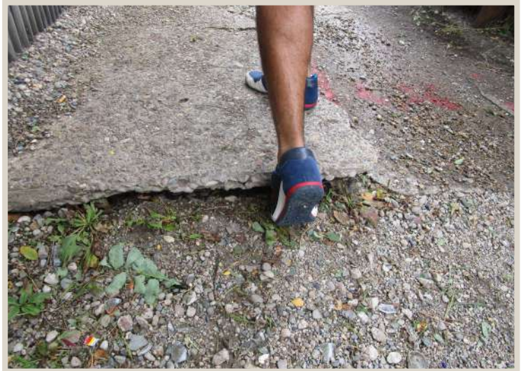
Figure 134. Sidewalks in extremely poor condition.
