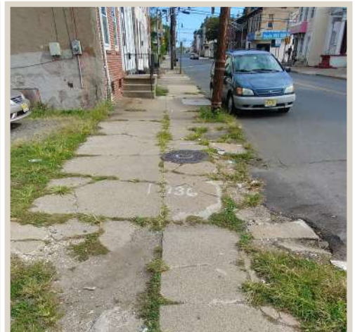
Figure 49. Vegetation growing along large cracks in the sidewalk.
