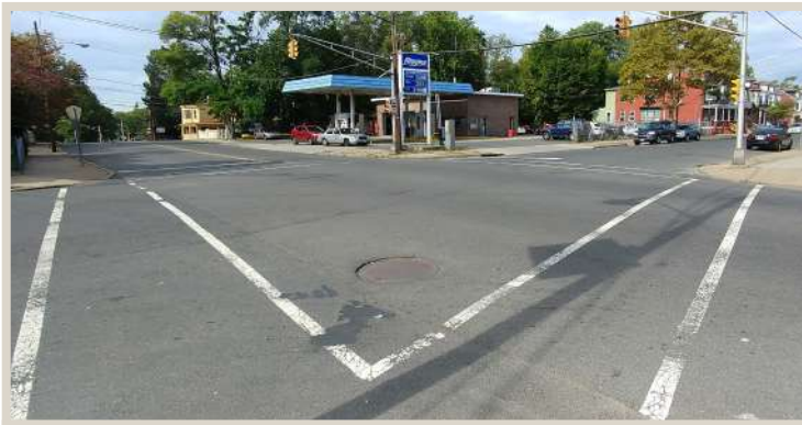
Figure 50. Intersection lacks pedestrian signals and ADA ramps.
