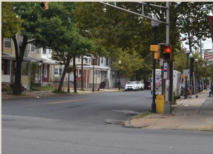
Figure 177. A missing crosswalk at the long intersection of Brunswick Avenue and N Olden.
