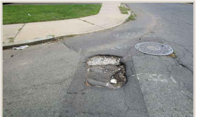
Figure 148. Asphalt near crosswalk in poor condition.
