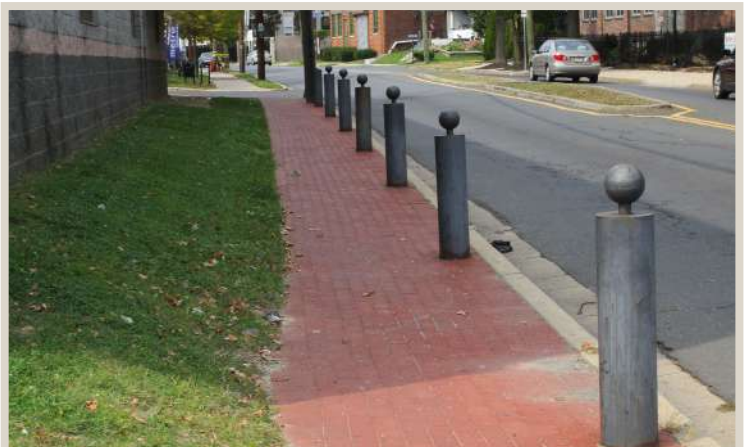
Figure 152. Sidewalk protected by bollards.
