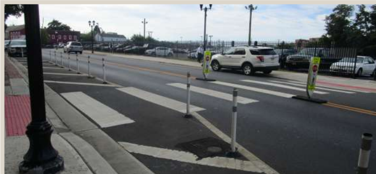
Figure 181. Ramps should direct pedestrian straight into the crosswalk as in this picture from South Broad Street.
