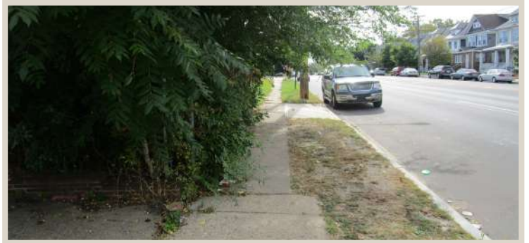
Figure 172. Overgrown bushes minimize usable sidewalk area.
