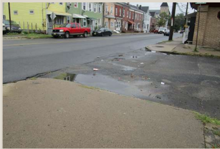
Figure 124. Missing crosswalk and non-compliant ramps.
