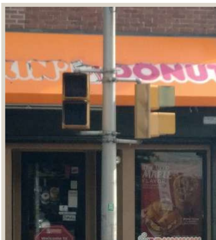
Figure 83. Non-functioning pedestrian signal
