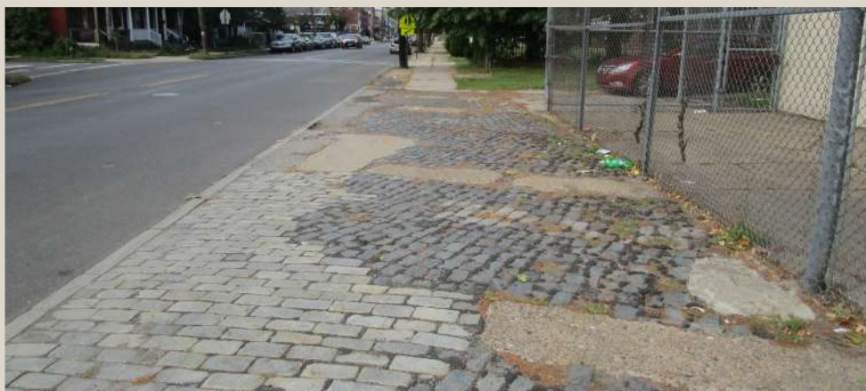
Figure 68. Uneven brickwork along East State Street.
