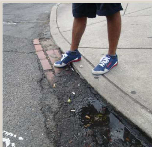
Figure 105. Compromised curb ramp.
