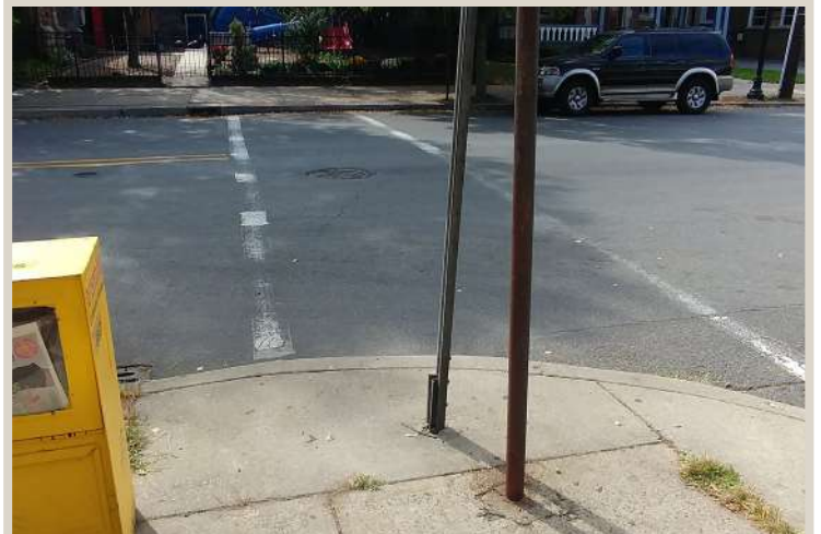
Figure 103. Missing curb ramps.
