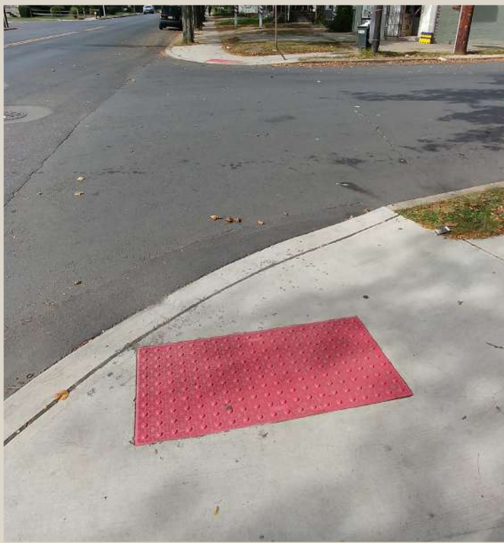
Figure 88. ADA compliant ramps, but missing crosswalks.
