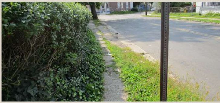
Figure 141. Overgrown plants blocking sidewalk.
