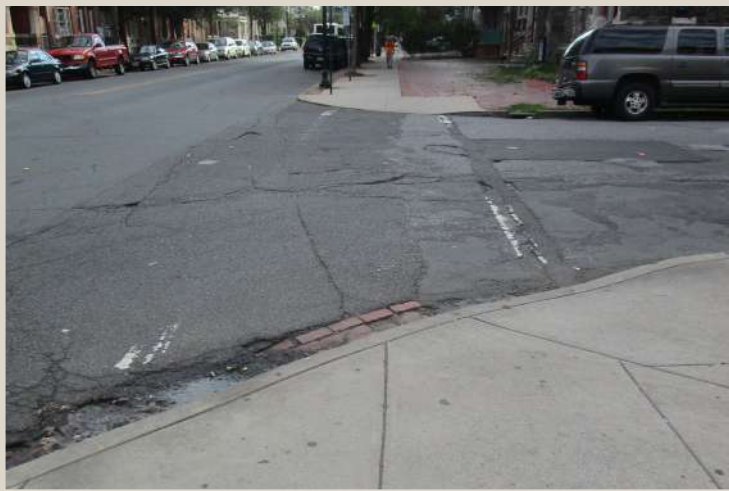
Figure 106. Faded crosswalks and non-compliant ramps.
