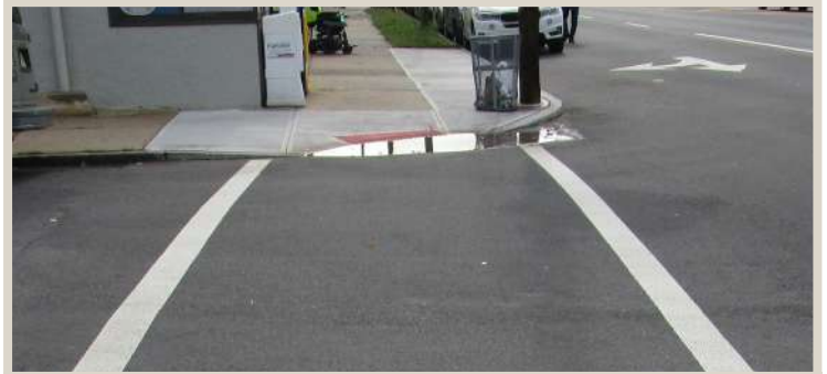
Figure 182. A curb cut which allows water to pool at the bottom is not usable.
