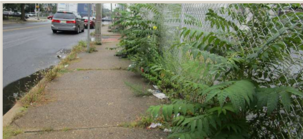
Figure 126. Overgrown brush blocking portions of the sidewalk.
