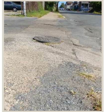
Figure 29. A sloping, uneven sidewalk.
