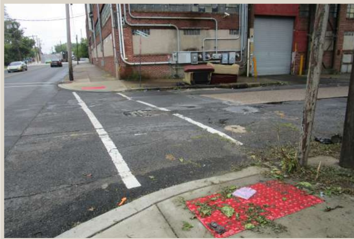
Figure 133. Grass clippings cover truncated dome across from abandoned building.
