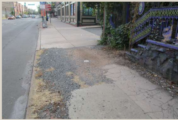
Figure 111. Sidewalk reduced to gravel.
