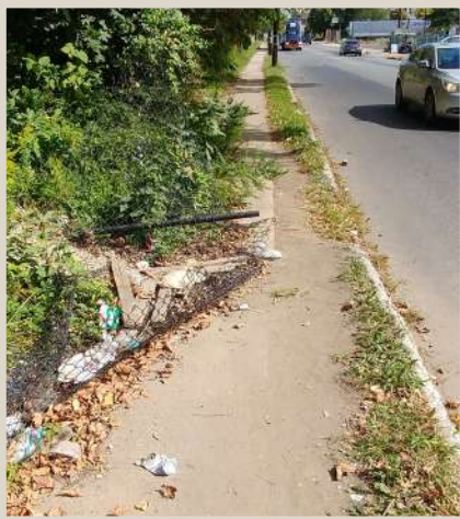
Figure 31. Fallen fence, litter and overgrown vegetation.
