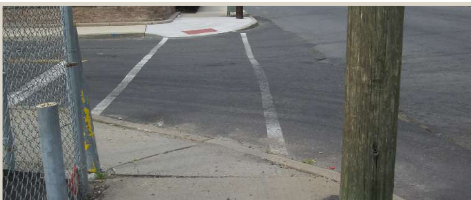
Figure 155. Non-compliant ADA ramp is oriented diagonally into the intersection.
