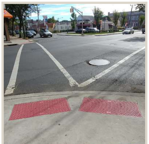
Figure 84. Non-functioning pedestrian signal.
