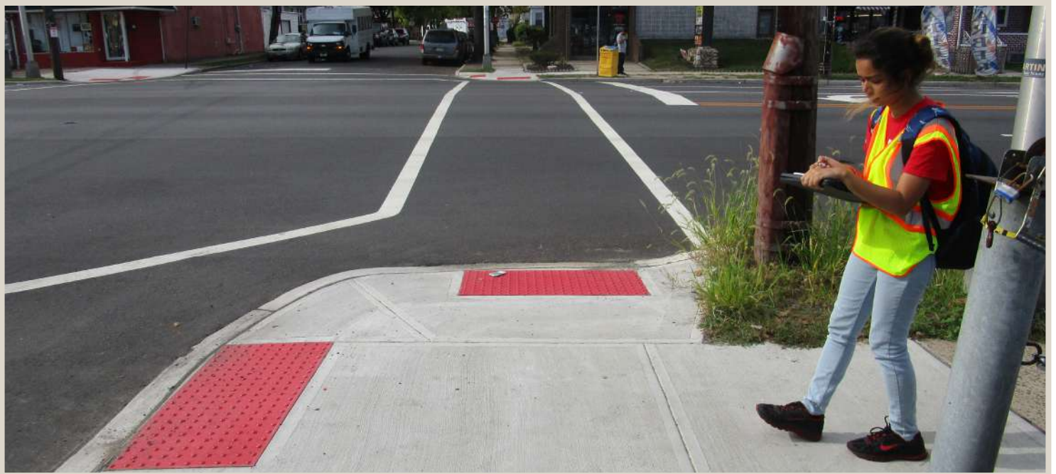
Figure 174. Sidewalks and ramps in excellent condition.
