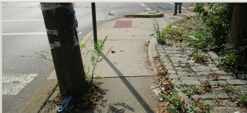
Figure 64. Utility pole drastically minimizes available walking space for pedestrians.
