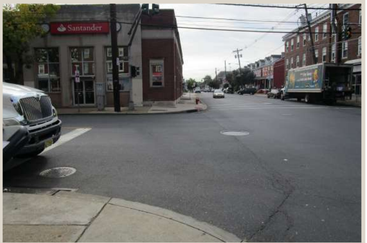
Figure 63. Missing crosswalk at North Olden Avenue intersection.
