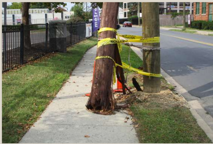
Figure 149. Haphazard utility pole work.
