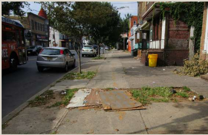
Figure 66. Missing sidewalk with makeshift bridge.
