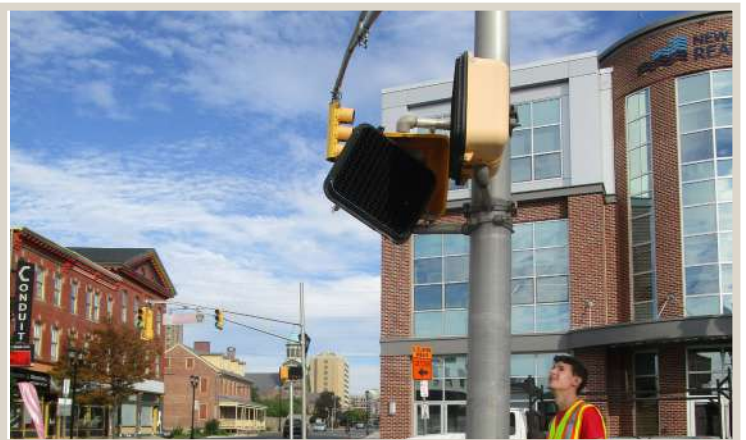
Figure 162. Non-operational pedestrian signal.
