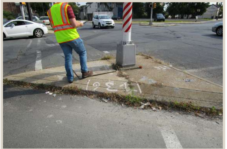
Figure 146. Missing ramps on pedestrian island.
