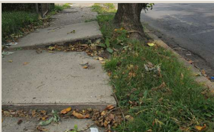
Figure 147. Roots have lifted the sidewalk into stairs.
